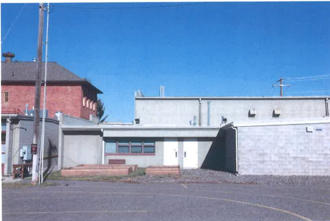
Feature #20 Facing: North
