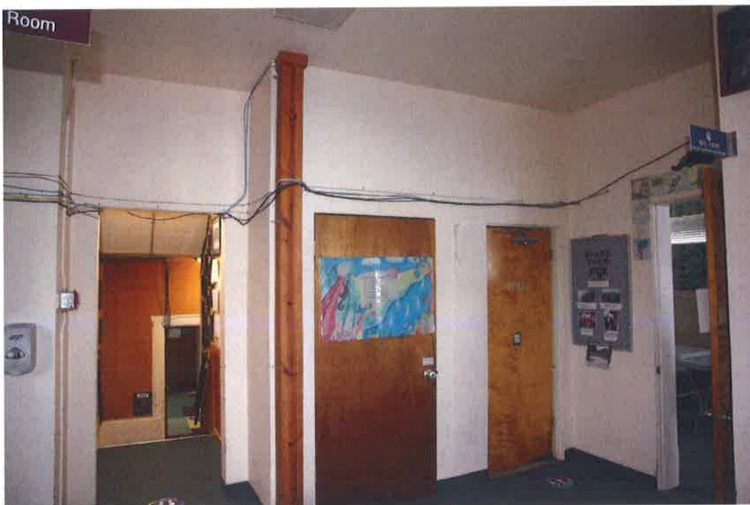
Feature #30 Description: Entry hall of 1915 Gallatin Gateway School. Facing: Southwest
