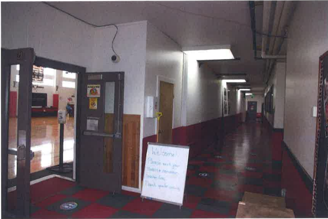
Feature #38 Description: Corridor between gym and classrooms of 1978 Gymnasium wing. Facing: Northeast
