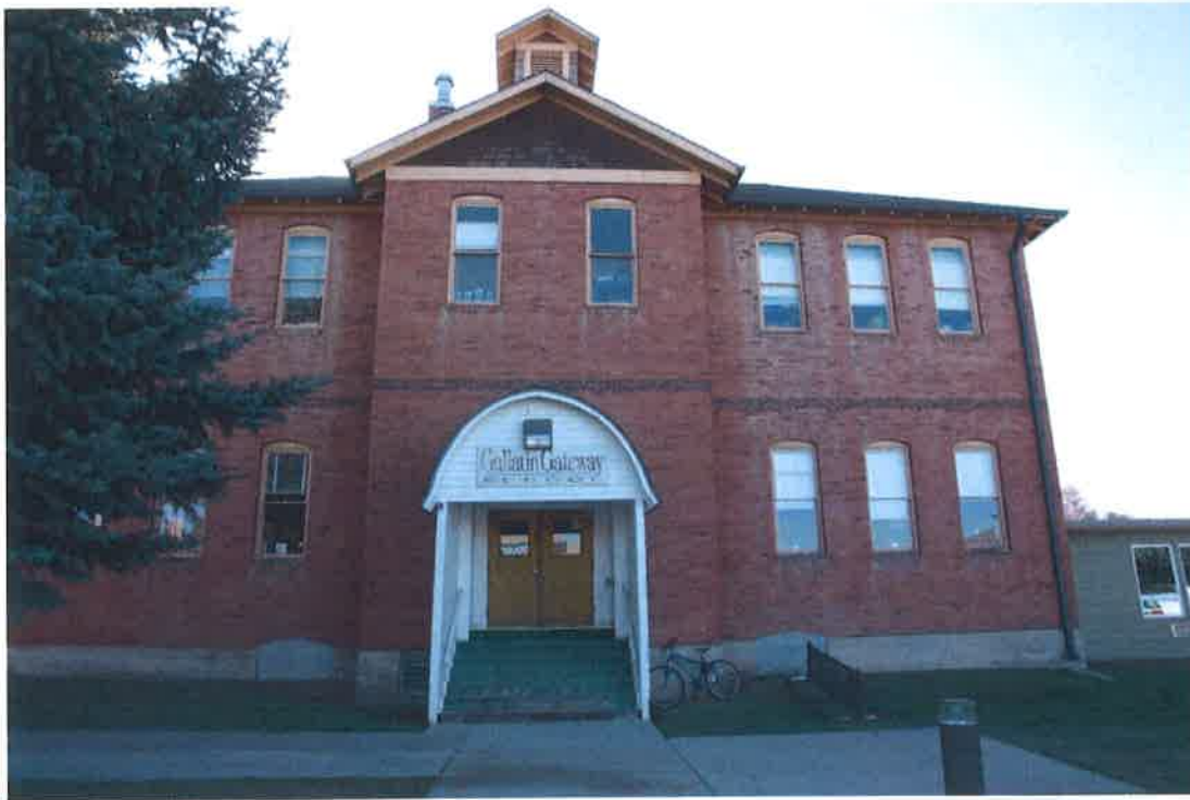
Feature #5 Facing: South
