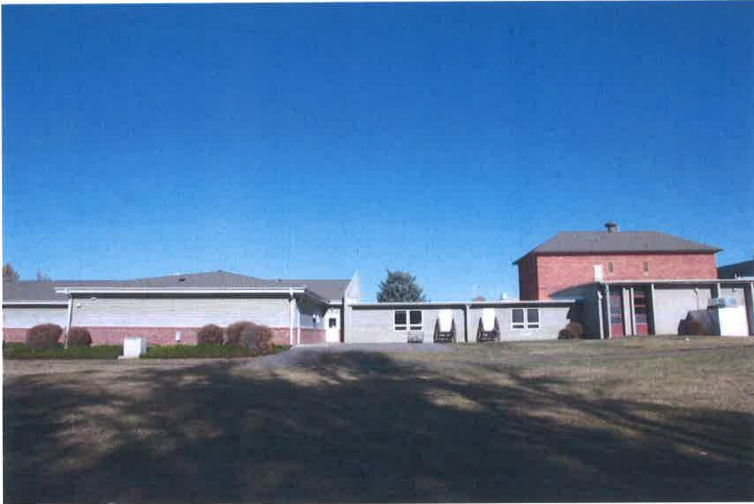
Feature #19 Facing: North
