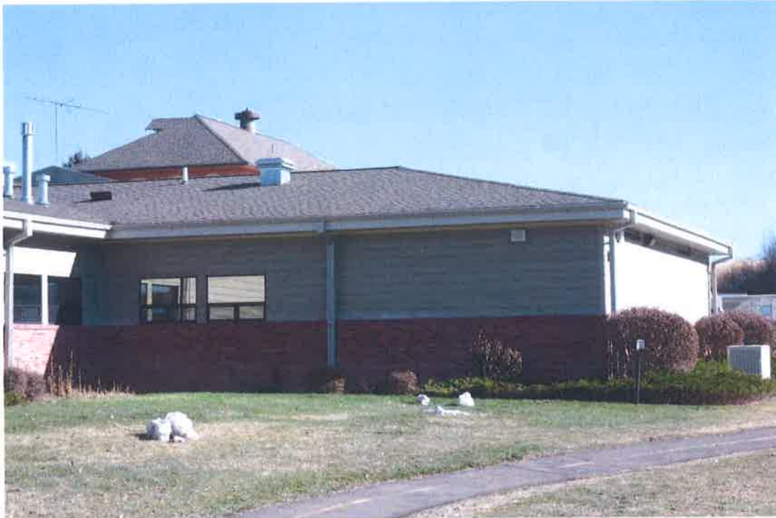
Feature #17 Facing: East
