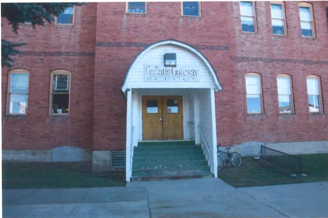
Feature #8 Description: North, entry façade of Gallatin Gateway School. Original 1915 building. Facing: South
