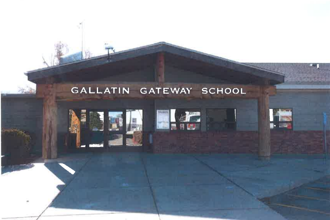
Feature #10 Description: North, front, façade of Gallatin Gateway School's 2002 entry. Facing: South
