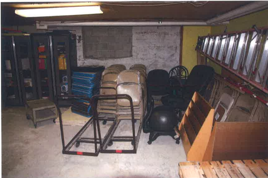
Feature #35 Description: East basement wall of 1915 Gallatin Gateway School. Facing: East
