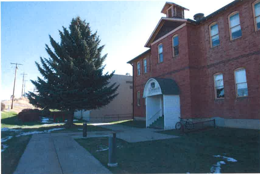
Feature #7 Description: North facades of original 1915 building at right, with 1978 gym beyond. Facing: East
