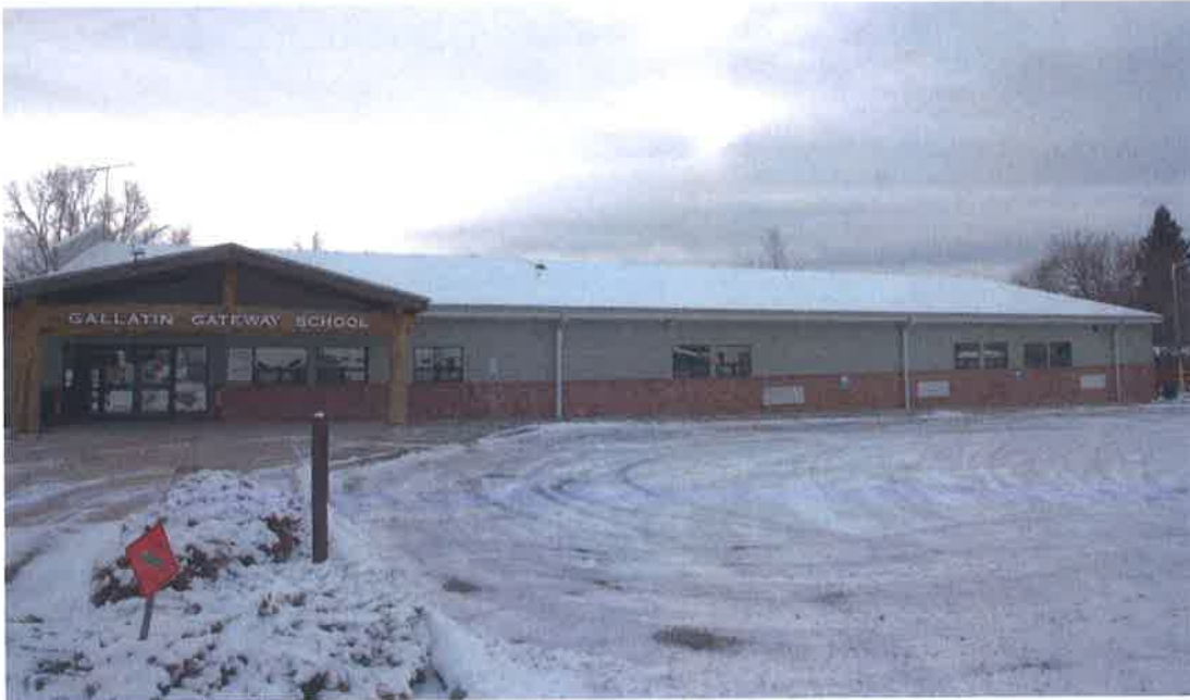
Feature #11 Facing: South
