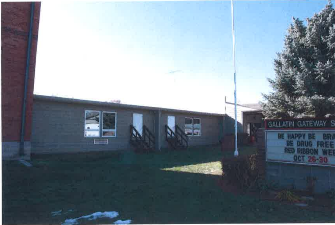
Feature #9 Description: North facade of Gallatin Gateway School. 1961 addition. Facing: Southwest
