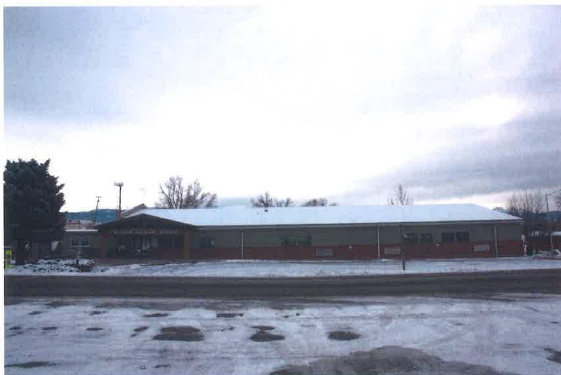
Feature #2 Description: North, front, façade of Gallatin Gateway School's 2002 wing. Facing: South
