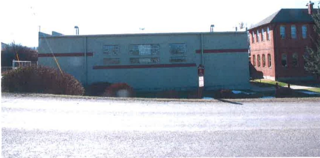
Feature #3 Facing: South
