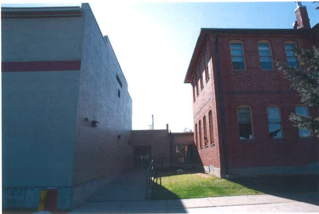
Feature #4 Facing: South
